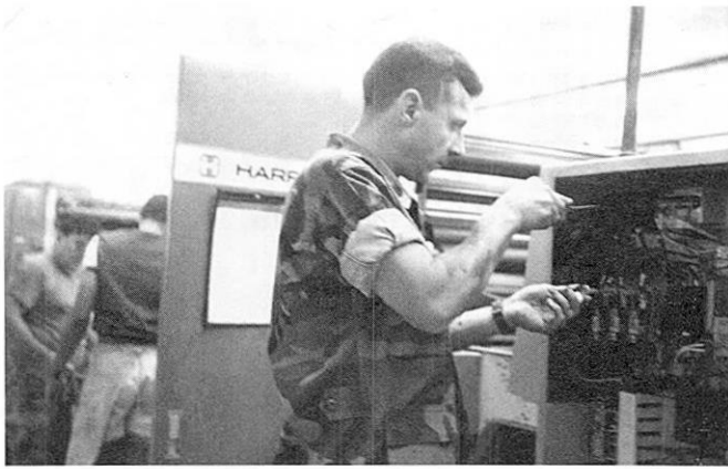
SSgt Tommy Williams starting to dismantle one of the six Harris LXG-FR offset printing presses that were removed from the press room in June to make room for Heidelberg SORD presses.
