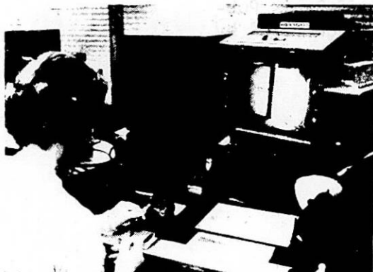
Original method: tape-slide teaching machines. They worked but took up a lot of bench space.
